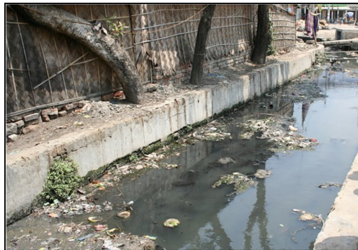
Open toilet near water
