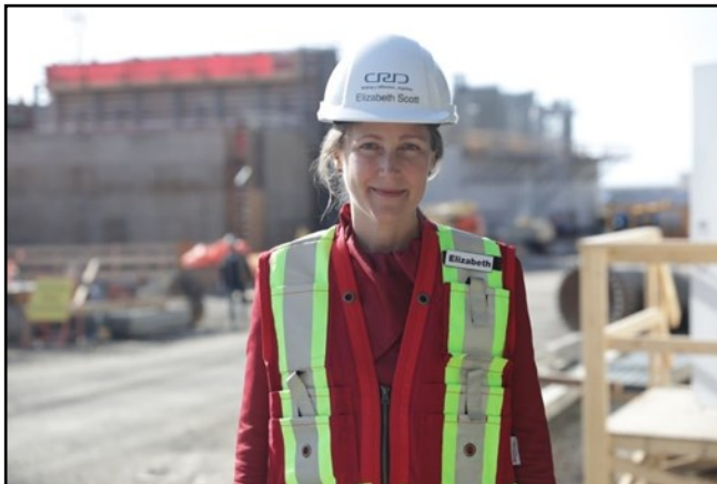
Deputy project director Elizabeth Scott says the most challenging part of the wastewater treatment project is that it requires laying as much as 30 kilometres of pipe, which will run through urban areas. (Briar Stewart/ CBC News )
